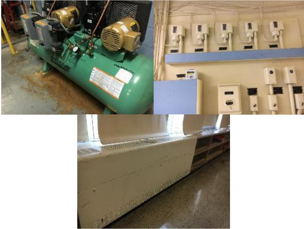
Figure 16-Pneumatic Control System
